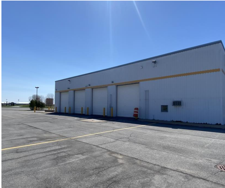
Exterior of Building
