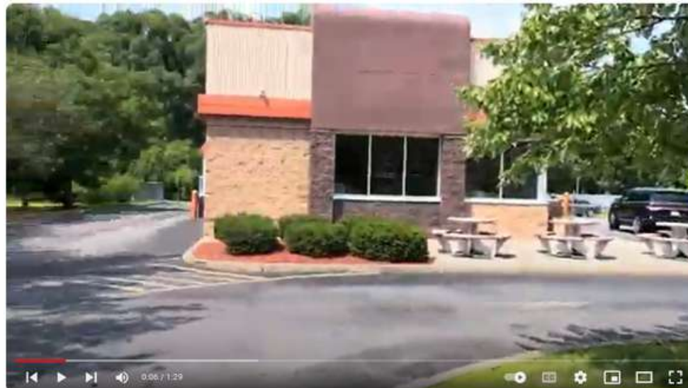
392 New Karner Rd, Albany, NY - Exterior Walk Through - Former Dunkin
